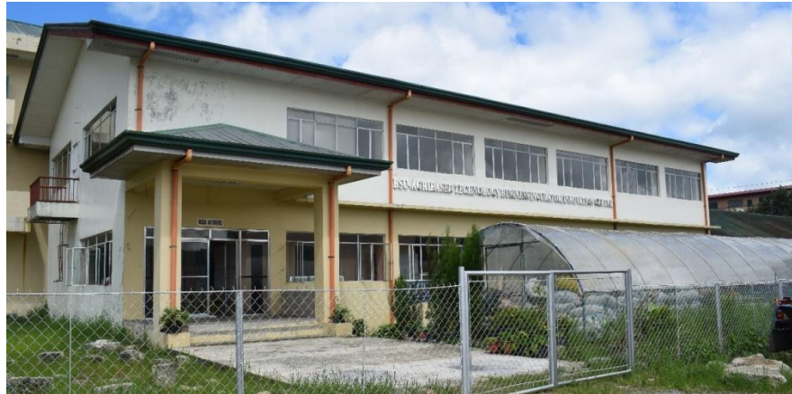
Plate 1. Main ATBI/IC building where the Co-Creation Lab is located at the second floor.
